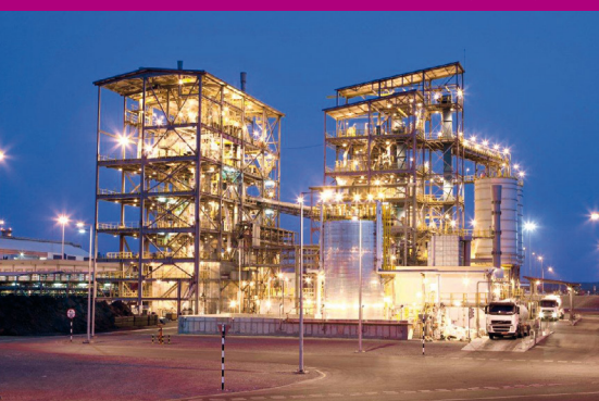
Green Anode Plant - Sohar Aluminium (Oman)
